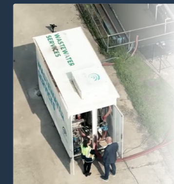
On-site special treatment applications
